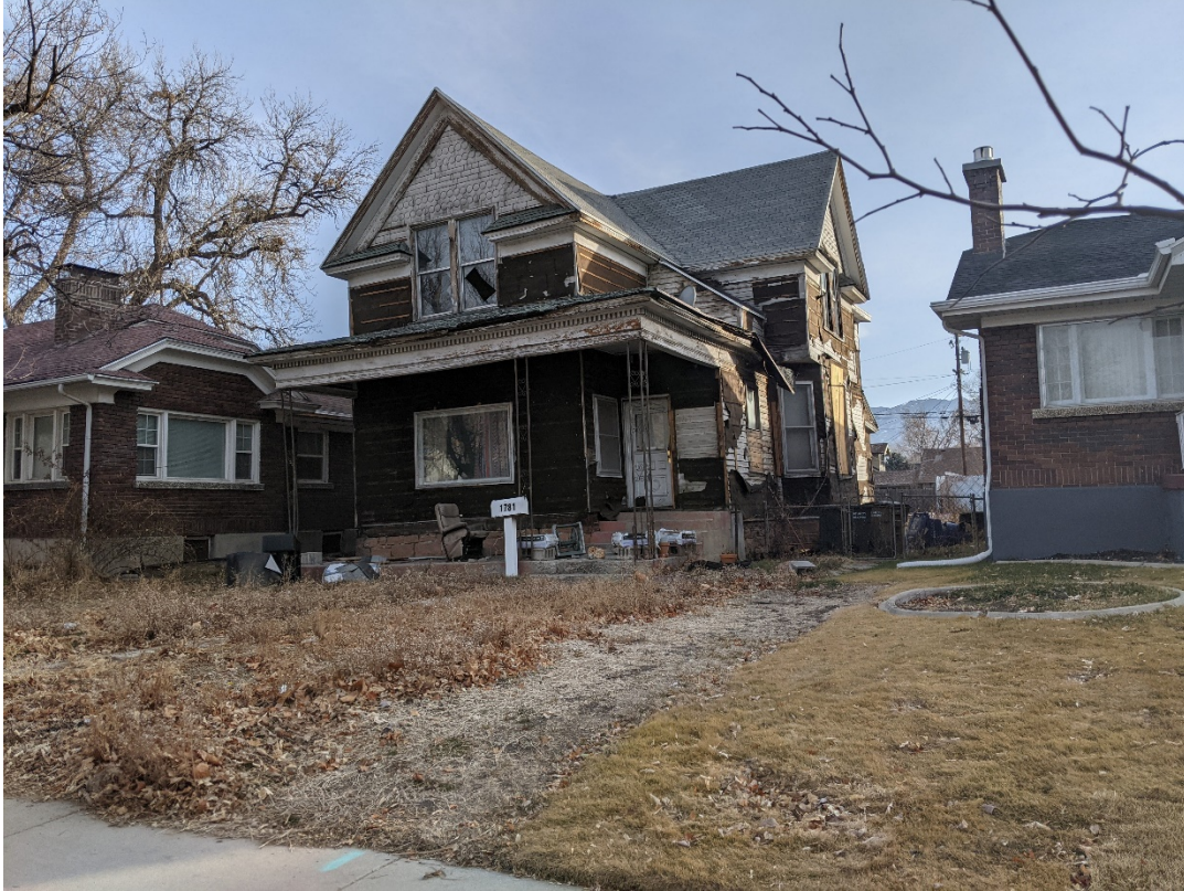
Figure 3 – The existing home on the property will be demolished and replaced.
